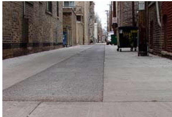
...with pervious paving
